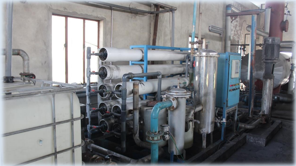
Figure-1: Reverse osmosis plant for preparing water for wet finishing processes and boilers
