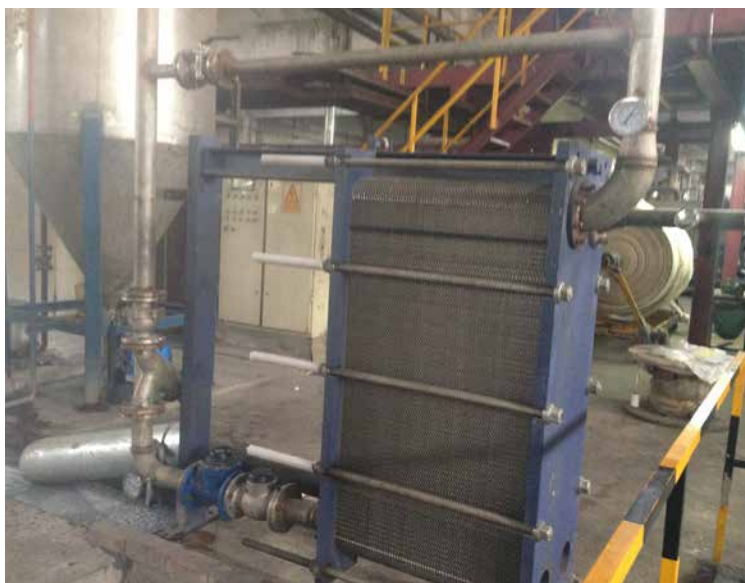
Figure-22: Plate heat exchanger for heat recovery from composite textile wastewater
