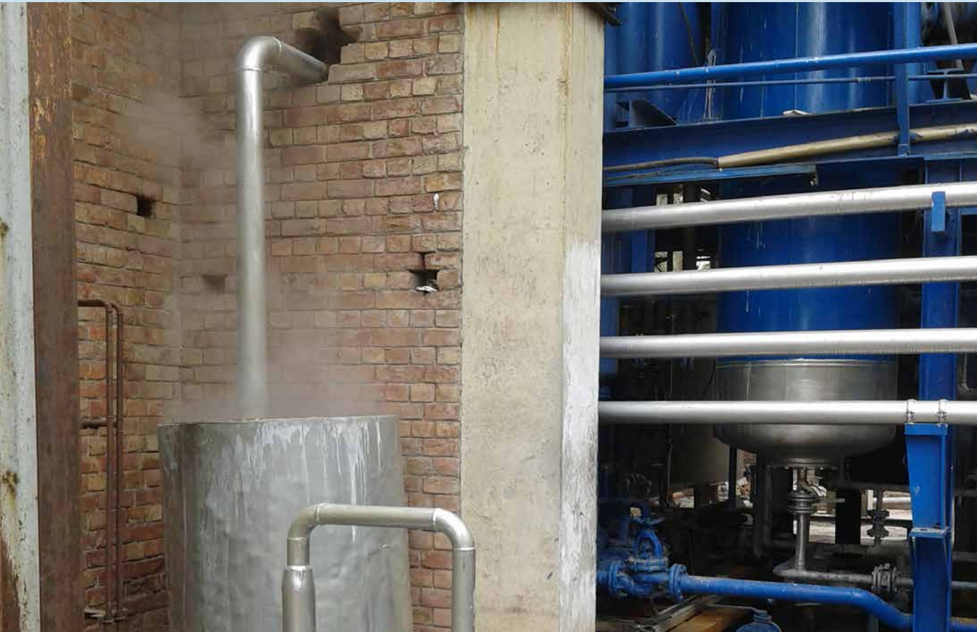
Figure-6: Vapor condensate from CRP is collected at over ground tank and then supplied to the pretreatment machine for post bleaching washing
