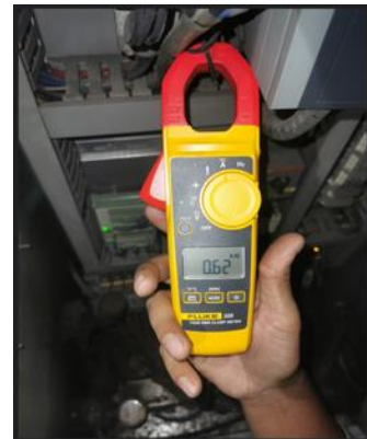
Measuring ampere of the dyeing machine.
